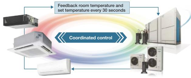
Calculate indoor refrigerant temperature and control the airflow automatically based on the difference between the setting temperature and actual indoor temperature. \* When fan speed is Auto.
